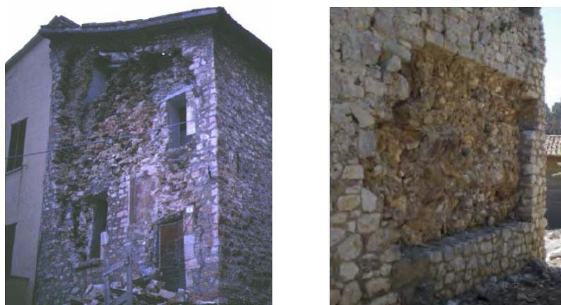
Figure 1.1: Failure modes of multi-leaf stone masonry walls [Modena *et al.* (2011)].
