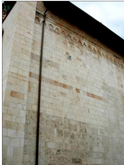
Figure 5.37: Damages corresponding to the results of the Flexural bowing of the façade. Diagonal crack on the west wall suggesting facade overturning (courtesy of EXPIN).
