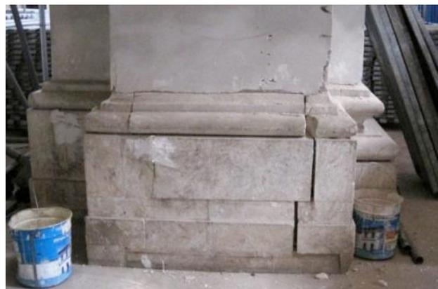
Cracking at base of columns
