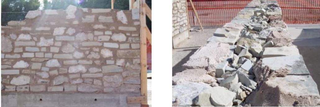
Figure 3.1: Building procedure: (a) Face of the wall; (b) Section with the rubble material.
