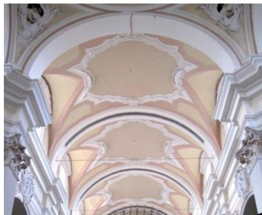
View of nave arches from transept, following some repairs including installation of temporary ties and FRP intrados reinforcing
